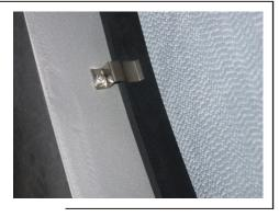
Systems in which sealing is not a main requirement use felt or rubber lip seals. These seals can be adjusted but they are not self-adjustable.
