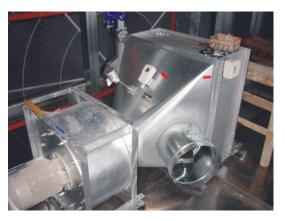
... and, through the connecting duct in the outgoing air section, blows it in the pulse chamber of the heat wheel in opposite direction of the exhaust air flow.
